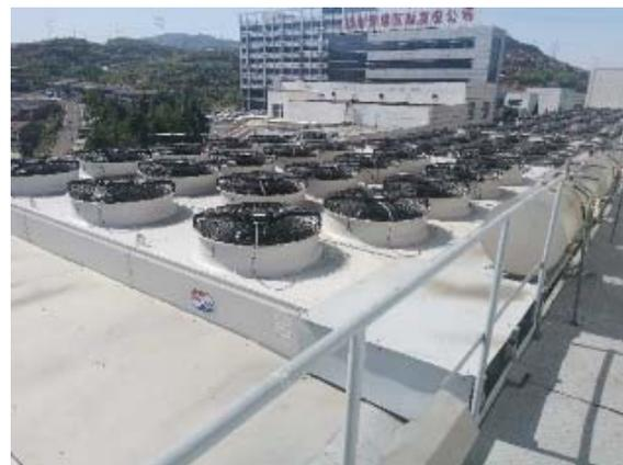
In June 2018, the retrofit was completed successfully, a before/after analysis was done and it showed that the new Güntner radiators was better. The main thermodynamic conditions had remained the same (e.g. heat dissipation consumption of the gen set, ambient air temperature, and inlet and outlet water
